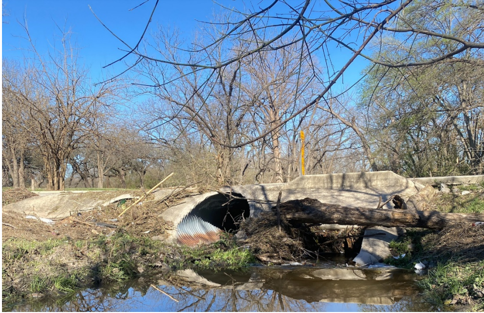
Figure 2 – Site Photo: McKie Street Crossing Upstream Face
