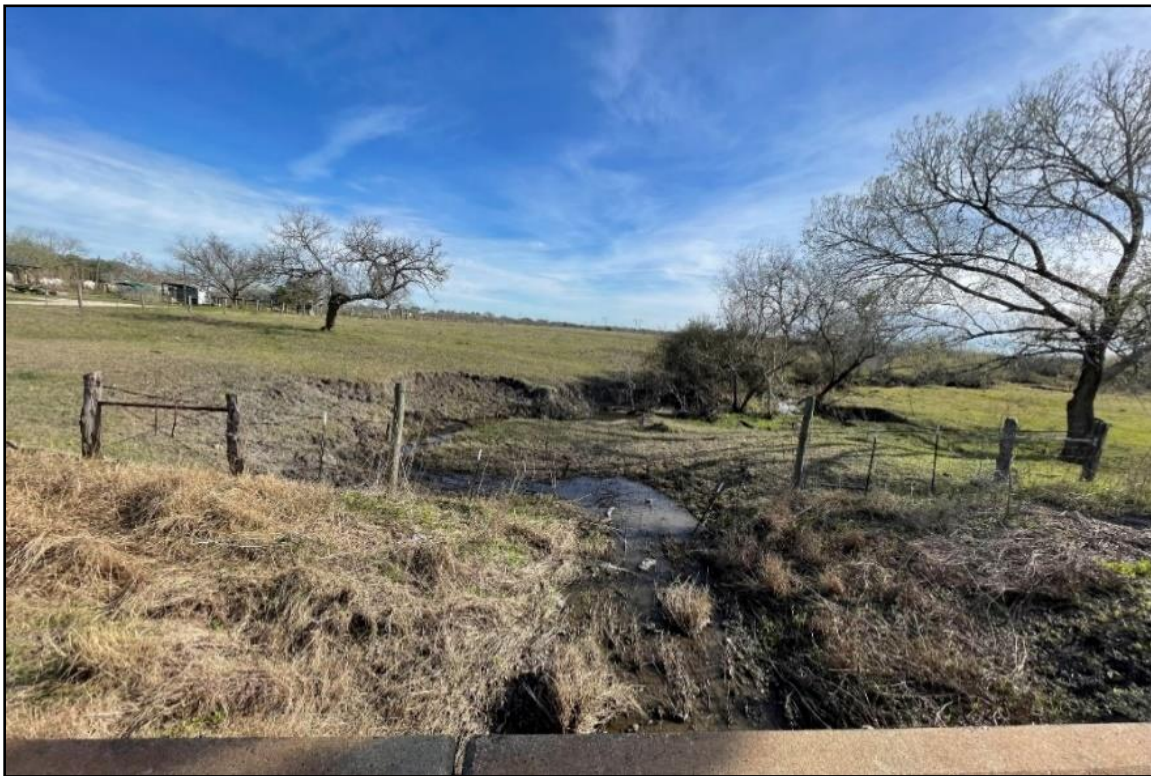
Figure 2: Downstream View at Nursery Road
