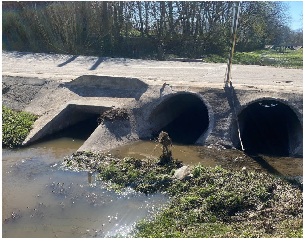
Figure 3 – Site Photo: McKie Street Crossing Downstream Face
